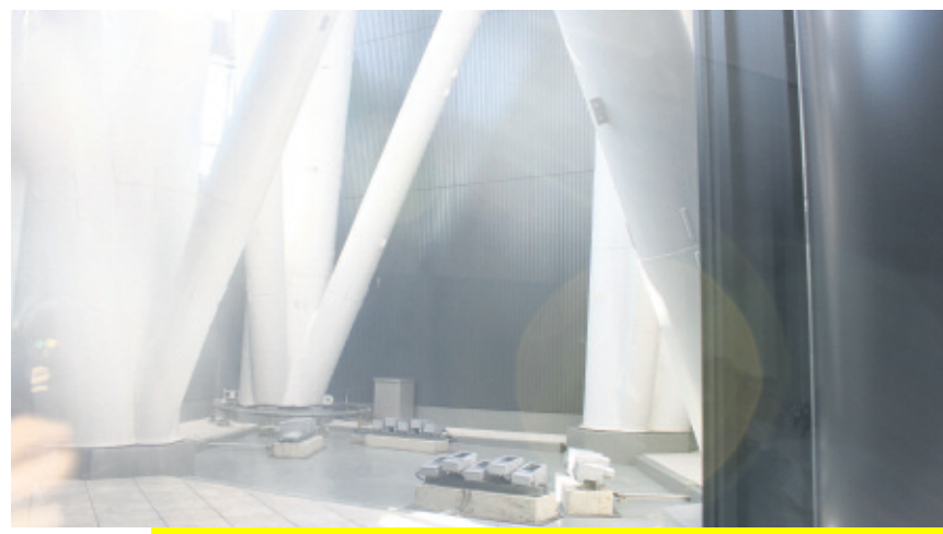
Massive steel tubes in Tokyo Sky Tree's core – an estimated 37,000 steel girders give strength to this tower.
